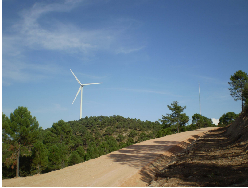
Figure 3: Wind turbine under test and reference mast used in the power performance measurement.
