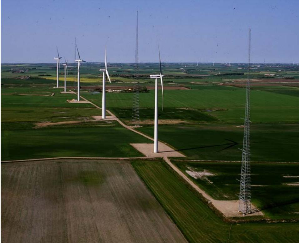
**Figure 2** The row of wind turbines at Høvsøre with the 116.5m meteorological tower in the foreground. The picture is taken from a low flying aircraft to the south-west of the mast..
