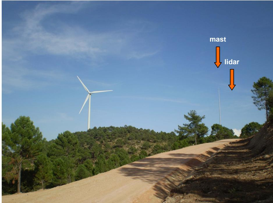
**Figure 5:** Location of meteorological mast, lidar and nearest wind turbine. Picture is taken from the West.
