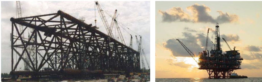
Figure 3: Petronius tower section under construction (left) and with topsides installed
