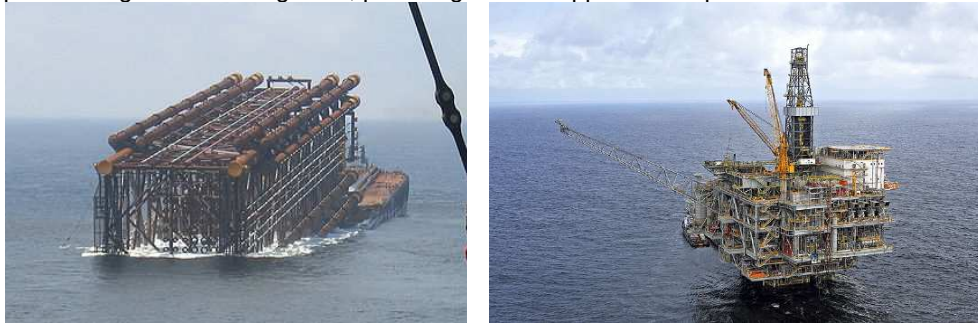
Figure 4: Benguela/Belize tower section during launch (left) and with topsides installed
