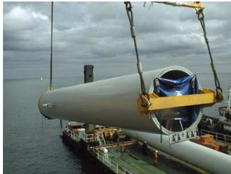
Figure 3.9: Lifting of a tower section for installation
