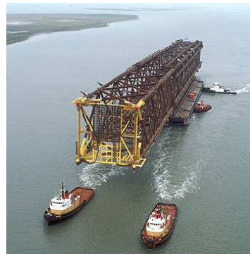
Figure 9.2: Baldpate platform in place (left) [9] and tower section during transport [48]
