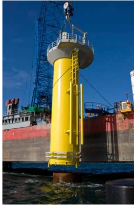
Figure 3.7: Transition piece installation [45]
