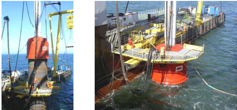
Figure 3.4: Pile driving at Offshore Wind Farm Egmond aan Zee
