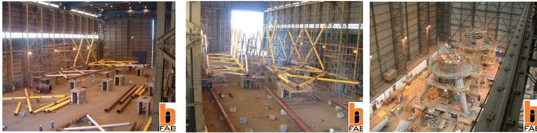
Figure 3.3: Various stages in the production of a jacket structure [44]
