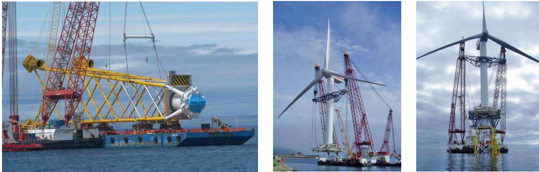
Figure 3.13: Various stages of the installation at the Beatrice demonstrator project [47]
