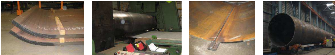
Figure 3.1: Rolling and welding of a foundation pile
