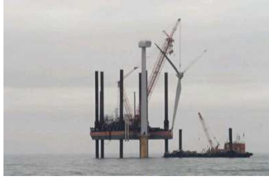
Figure 3.10: Installation of a rotor in one piece
