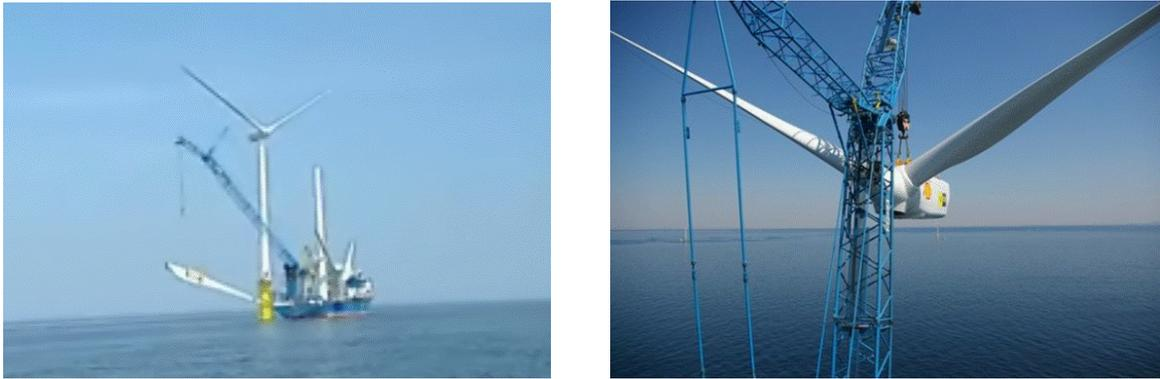
**Figure 22:** *Various stages in the installation of a turbine using the bunny-ear method*
