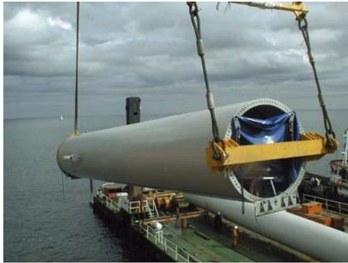
**Figure 20:** *Lifting of a tower section for installation*
