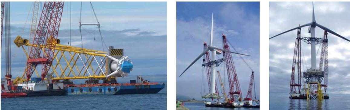
**Figure 23:** Various stages of the installation at the Beatrice demonstrator project
