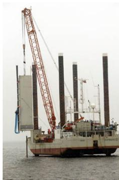
**Figure 18:** Transition piece installation
