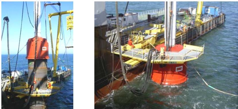
**Figure 15:** Pile driving at Offshore Wind Farm Egmond aan Zee
